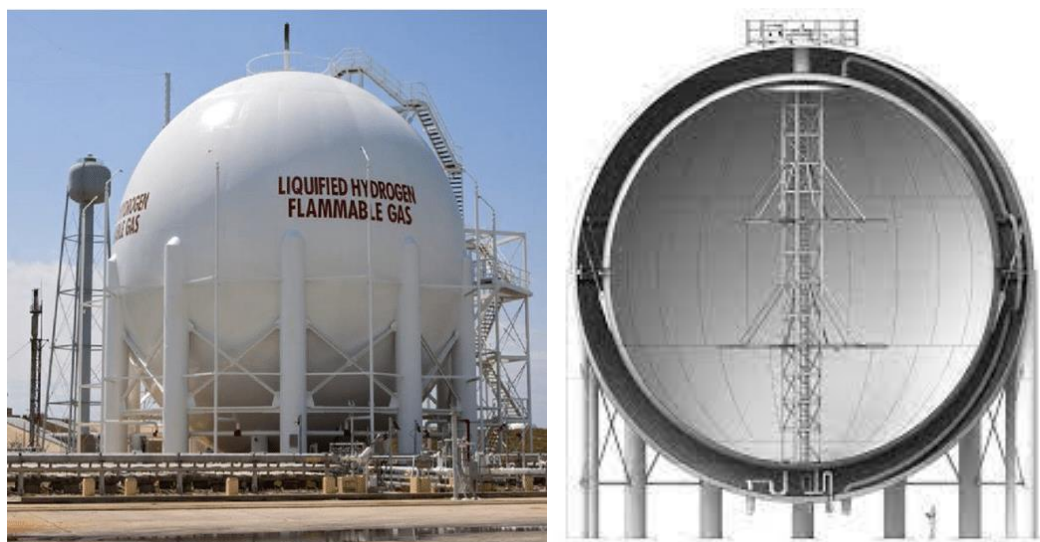
Figure 17. Large-scale spherical liquid hydrogen storage tanks employed by NASA 16 .
