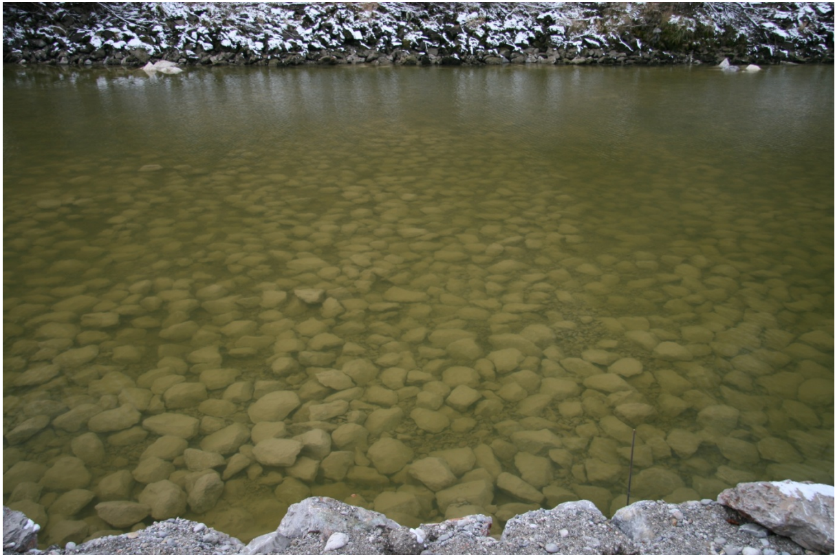
Figure 12: Stone cover of the river bed/rip rap as a bed protection against erosion
