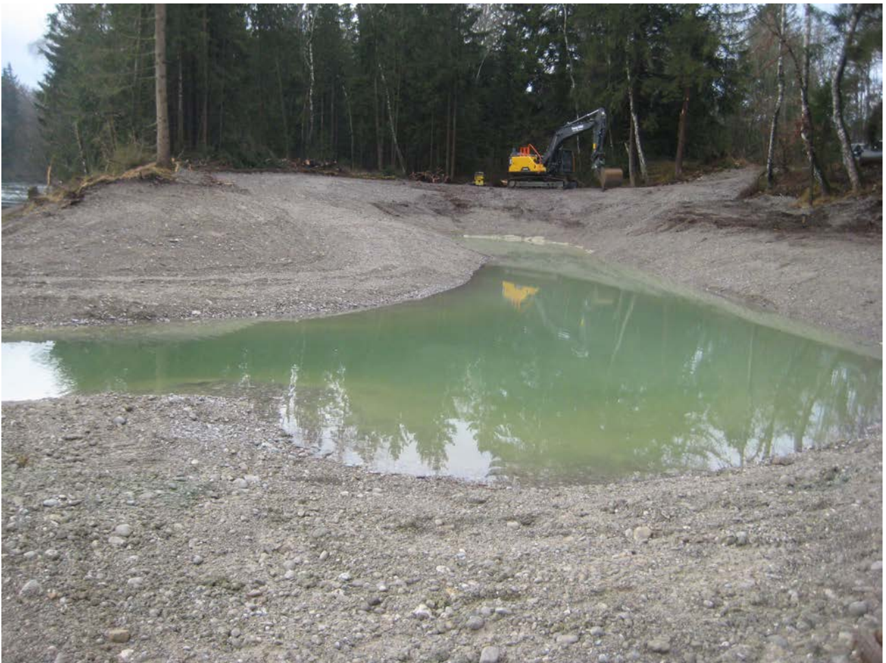
Figure 5: Artificial oxbow near Scheuring on November 30th the introduction of logwood debris and roots will be made soon.
