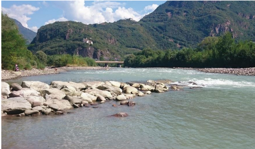
Figure 7 - Example of a flow deflector placed downstream the Roma bridge. View from downstream
