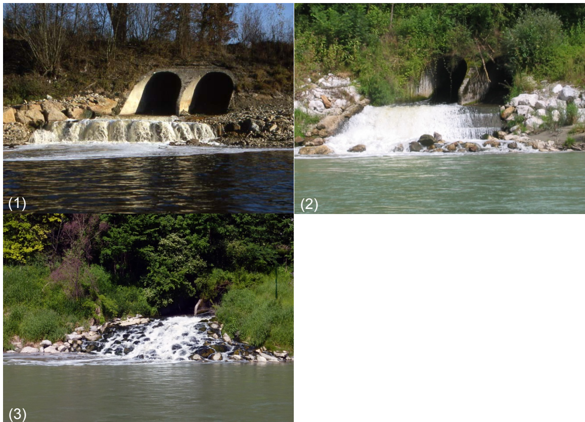
Figure 8: Inlet structure of the water treatment plant Siggerwiesen (km 58,4) Nov. 1986 ( Q = 90 \text{ m}^3/\text{s} ) (1); August 2004 ( Q = 200 \text{ m}^3/\text{s} ) (2); May 2017 ( Q = 288 \text{ m}^3/\text{s} ) (3)
