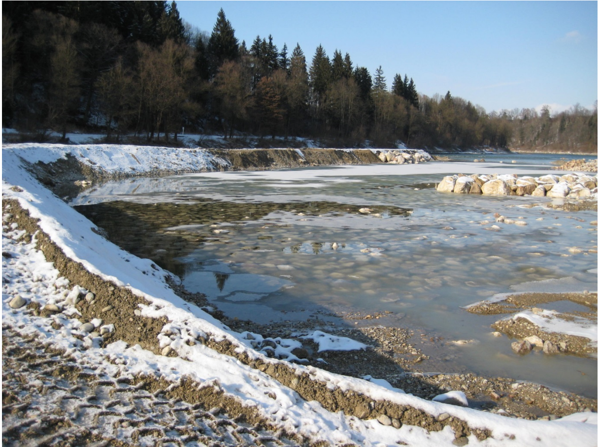
Figure 11: Construction of the rip rap during winter time (low flow period)
