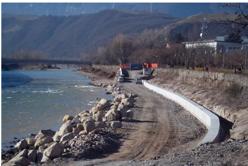
Figure 6 – Bank reinforcement through concrete kerb
