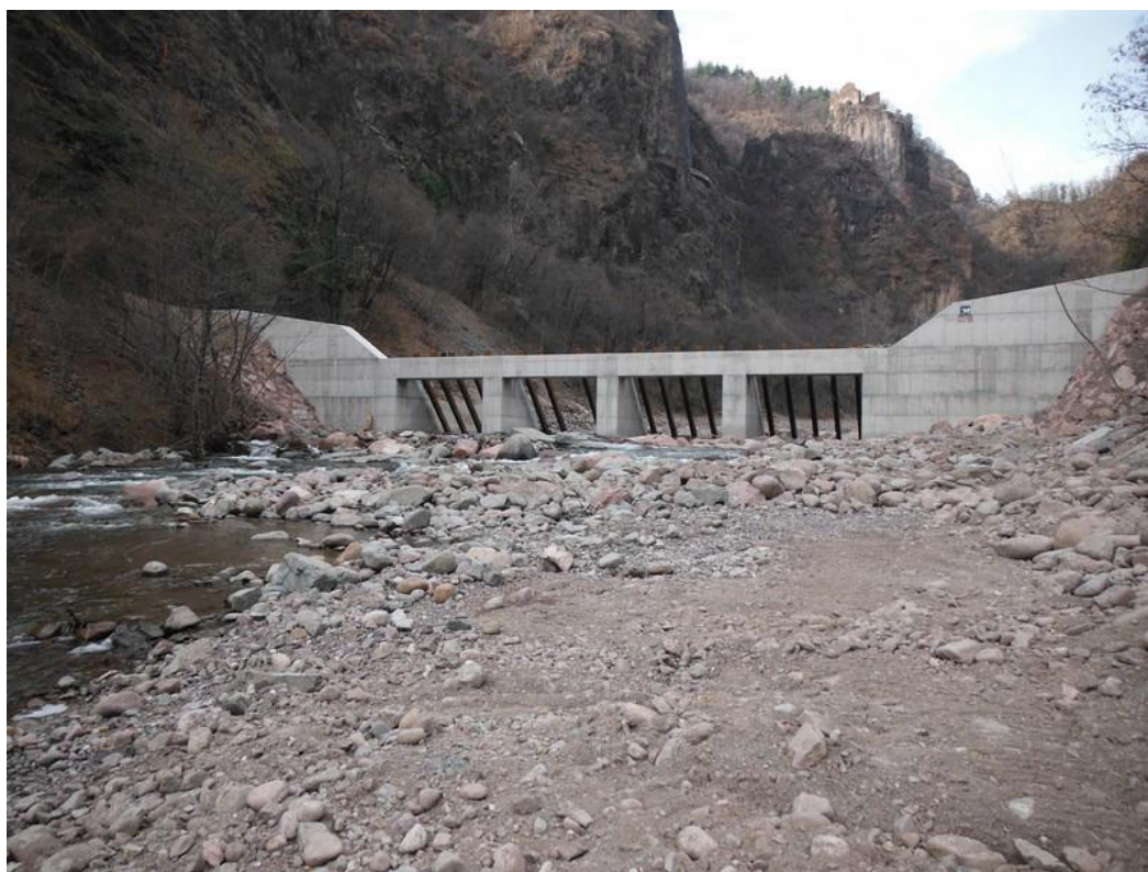
Figure 9 - Retention check dam constructed within the HyMoCARES project, sited 4.1 km upstream from the Isarco confluence. View from downstream to upstream
