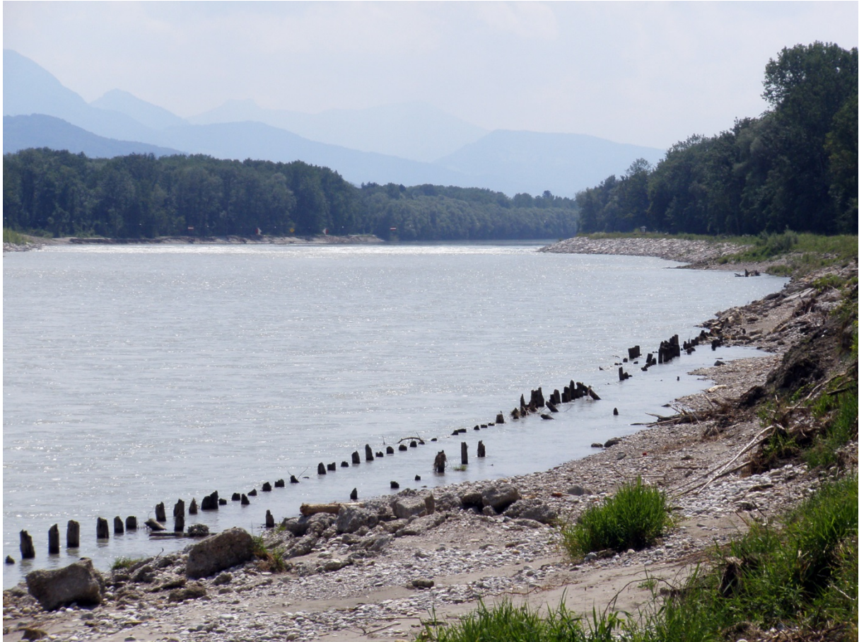
Figure 16: Salzach km 51,9, upstream view, bank erosion and old bank protection
