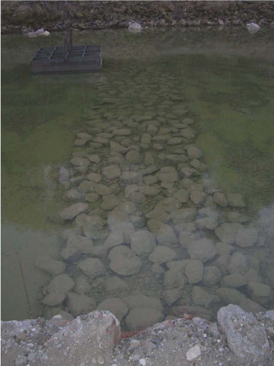
Figure 10: Construction of the rip rap by an evenly spaced stone cover
