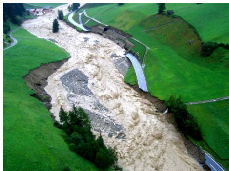
Fig. 27. Damages along Trisanna River after extreme flood (source: Baubezirksamt Imst).
