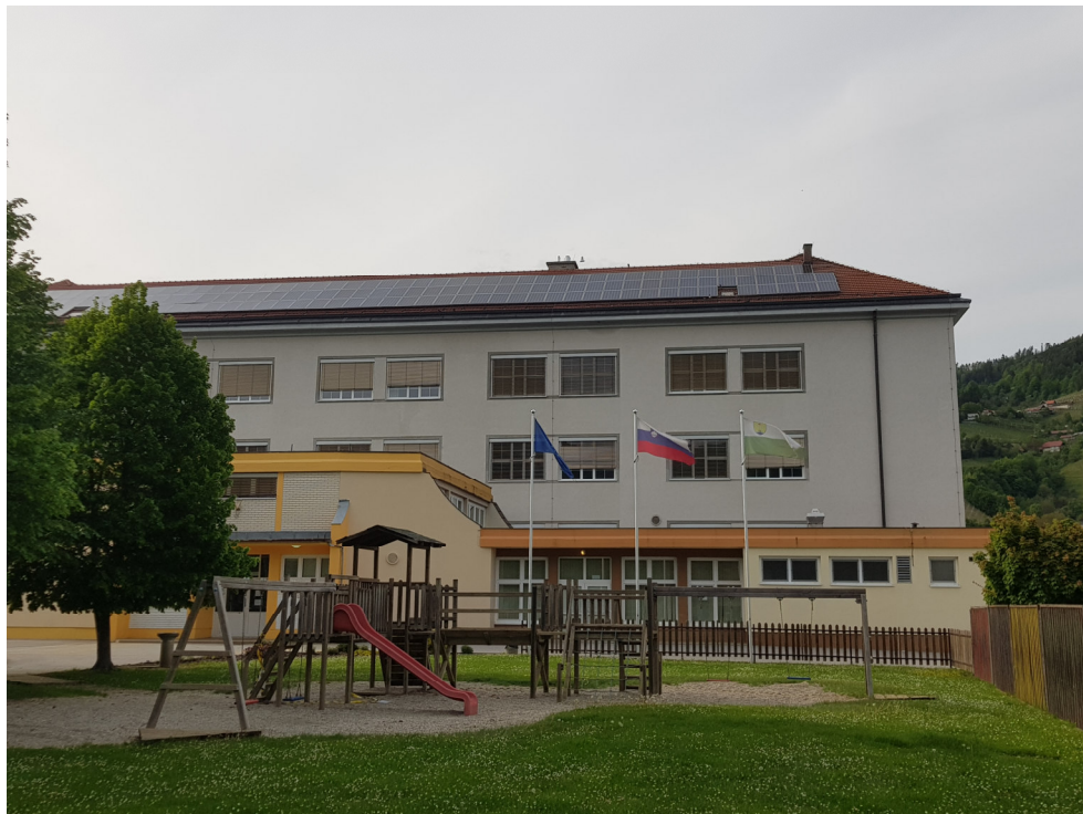
Figure 27 - PV installation on the south-oriented part of the roof of the school building roof (Selnica)
