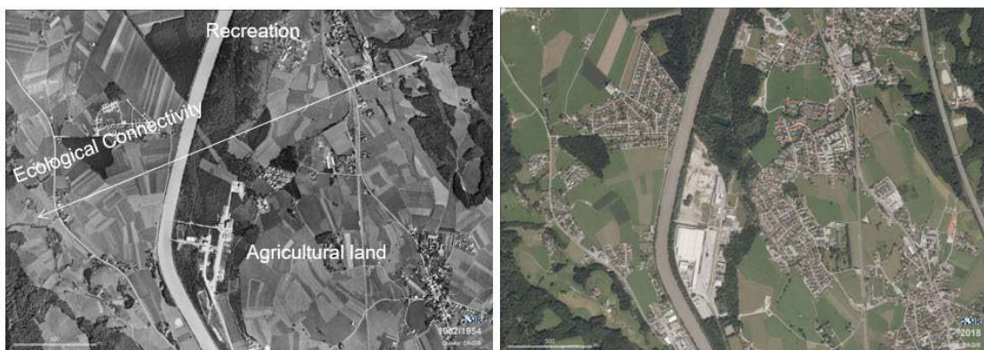
Figure 6: Settlement development 1953-2017 Oberalm (Tennengau/AT) – caused by the urban sprawl of the city of Salzburg
