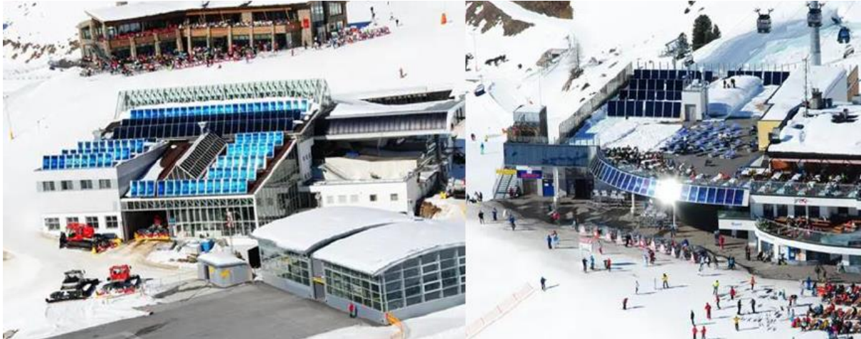
Figure 11: Solar PV installation for chalets and huts electrical demand in Austrian ski resort Ischgl [19]
